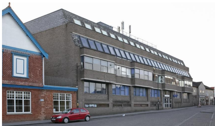
Figure 11 – Sulby House, North Street, Sudbury
