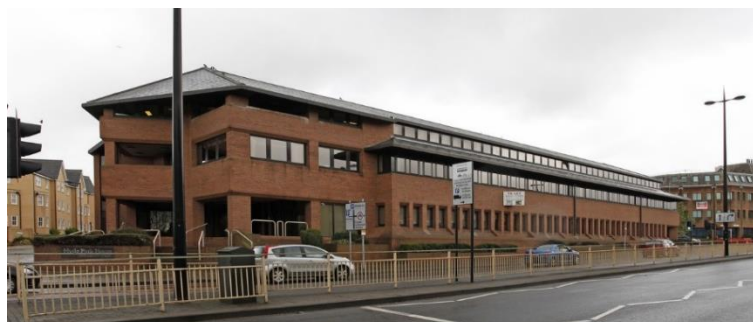
Figure 12 – Hyde Park House, 1 Crown Street, Ipswich
